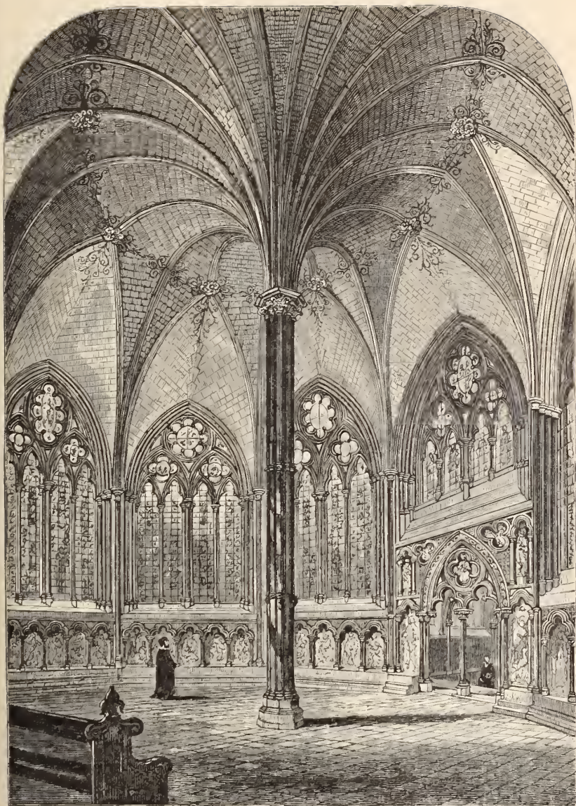
THE CHAPTER HOUSE AS RESTORED BY SIR GILBERT SCOTT.
